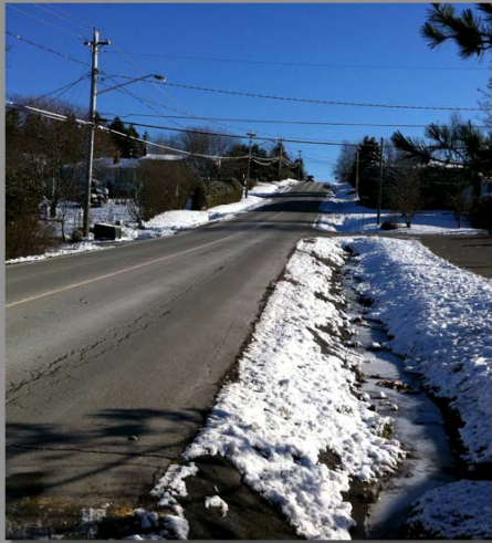
Many Qusipamsis streets are steeply sloped and/or have ditches that will require upgrades to allow the placement of AT infrastructure.
