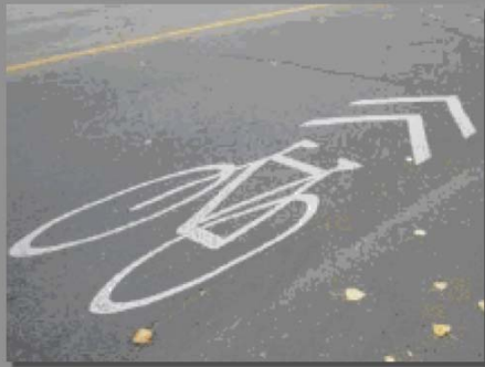
The "Sharrow" is a painted street graphic that incorporates the bicycle and directional arrow to indicate the shared nature of chosen corridors.
